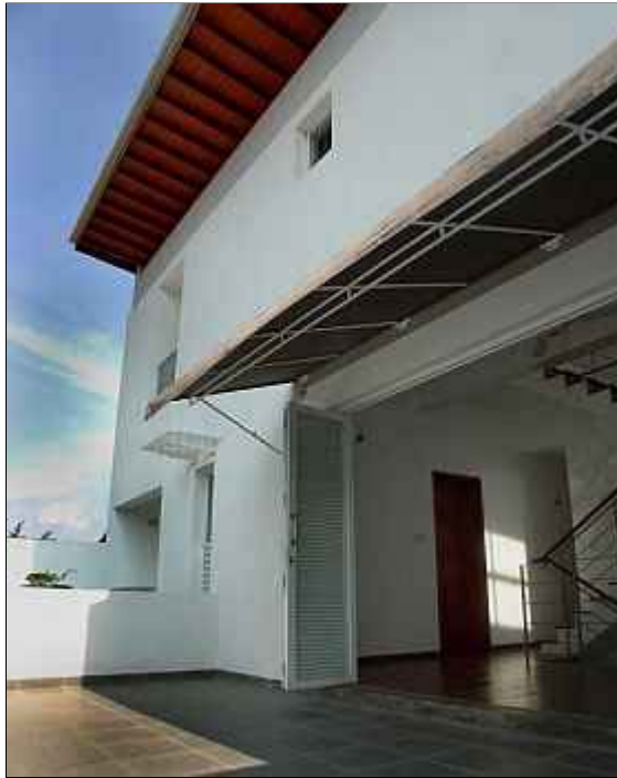
Twin Houses, Colombo. His architectural designs are always eco-friendly. The homes he builds are full of light and air.
